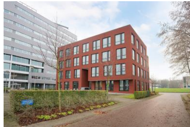
Pilot site 4: 4-stories building, Delftechpark
